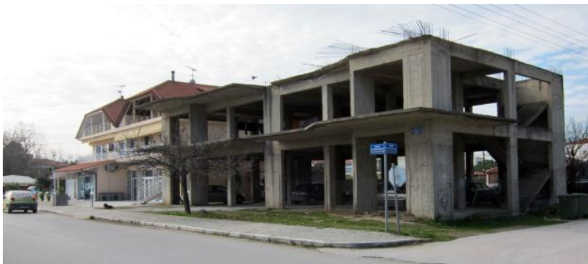
Picture 4. Construction without building permit
