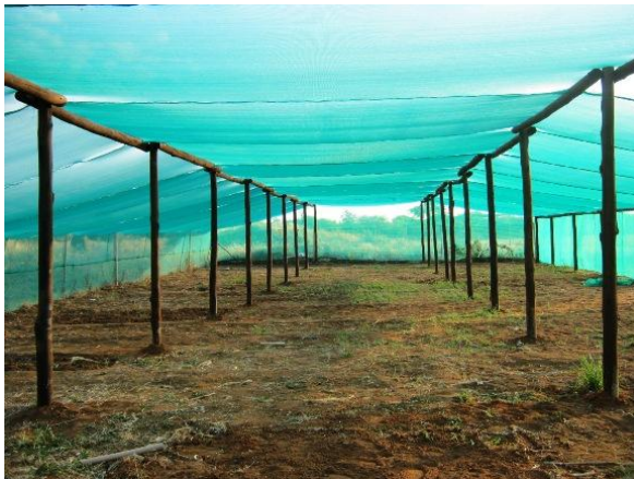
Figure 3: Fixed Net on the poles
