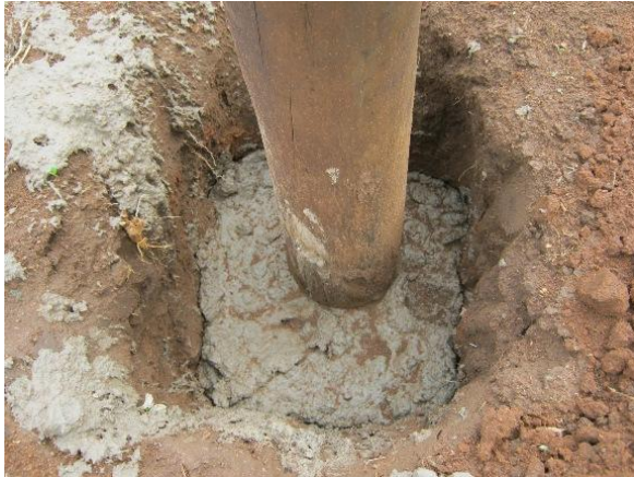
Figure 1: Fixing poles with cement and concrete
