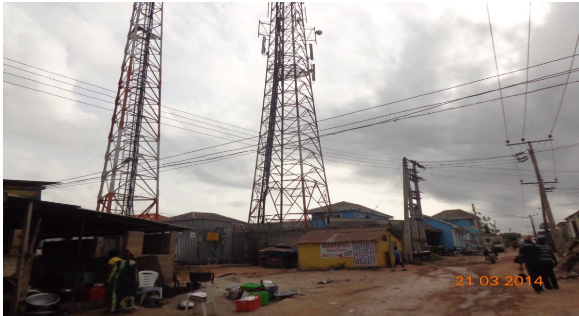
Plate 2: A photograph of the cell tower considered.
